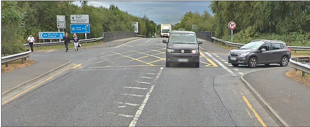
Figure 2.29: Vulnerable Road Users at Junction 7 (©2024 Google)
