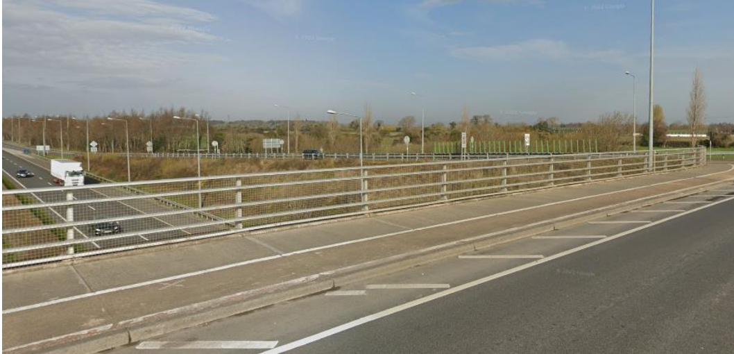
Figure 6.12: Segregated Vulnerable Road User Facilities on western side of existing structure (© Google Imagery ©2024 DigitalGlobe)
