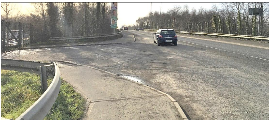
Figure 2.28: Junction 7 - Barton Transport Entrance (Arup Site Visit 5 th of February 2020)
