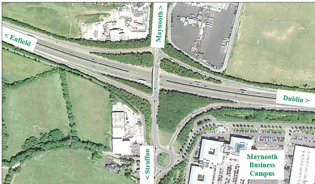
Figure 2.14: Junction 7 Maynooth – Aerial (© Google Imagery ©2024 DigitalGlobe)
