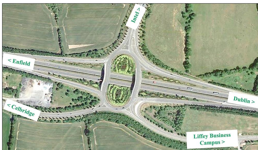
Figure 2.12: Junction 6 Celbridge – Aerial (© Google Imagery ©2024 DigitalGlobe)
